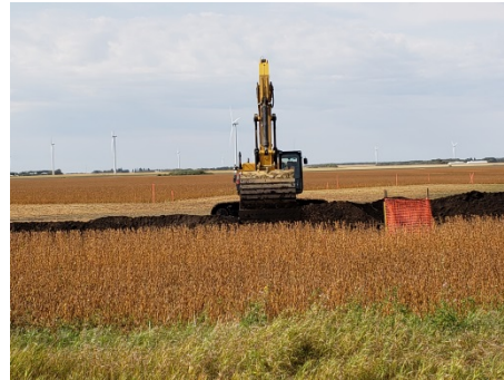
Sept 8/18 Photo facing West SF 48 West side of road across from St Leon station Excavator stripping edges of ROW.
