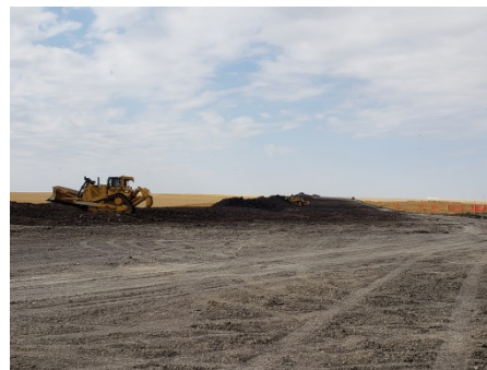
Sept 7/18 Photo facing West SF 43 (KP981+225) Dozers stripping and piling top soil.
