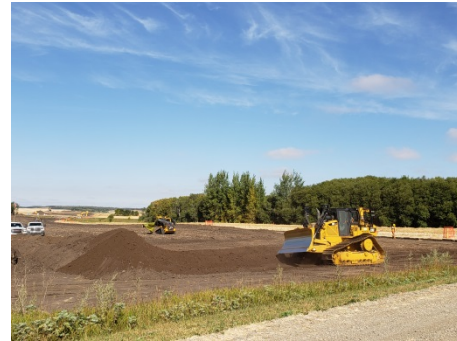
Sept4/18 Photo facing North West – SF 38A Dozer removing the improper soil that was used for the approach
