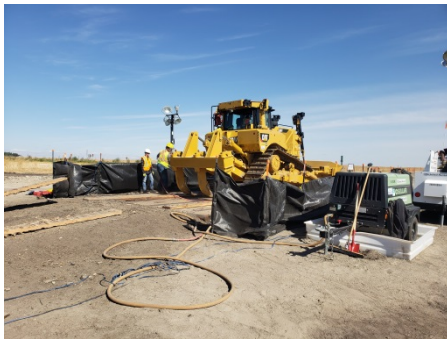
Sept4/18 Photo facing North East SF 37A cleaning station Dozer being sprayed with compressed air.
