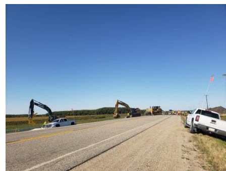
Sept 5/18 Photo facing South West – SF 41 Equipment crossing Hwy 23
