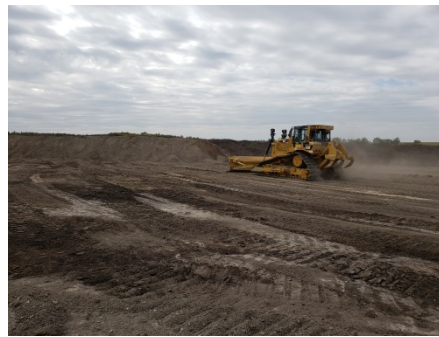
Sept 7/18 Photo facing South West SF 40A (KP978+140) one dozer piling top soil on the South side of the ROW
