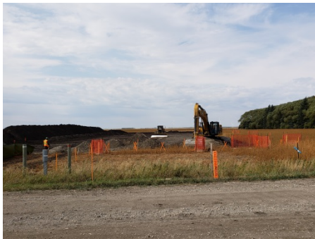
Sept 8/18 Photo facing West SF 43 (KP996+383) Excavator and dozer working to strip the edges of the ROW and build an approach.
