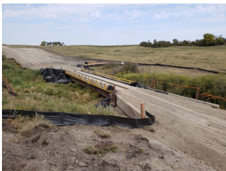
Sept 7/18 Photo facing North West SF 40A (KP978) Bridge installed at creek crossing.
