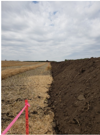
Sept 6/18 Photo facing West SF 39 West side of Hwy 34 Top soil piles within boundary line
