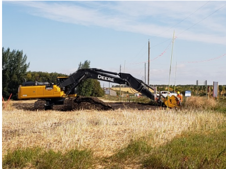
Sept4/18 Photo facing North - SF 39 Excavator stripping the edges of the ditch line
