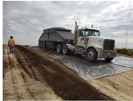
Sept 6/18 Photo facing South East SF 39 Gravel being laid out of tandem truck
