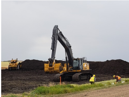
Sept 8/18 Photo facing SE SF 43A east side of road Crew laying out CAEPLA cloth, dozer piling soil
