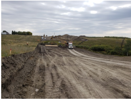
Sept 6/18 Photo facing East SF 40A (KP978) Bridge being installed at creek crossing
